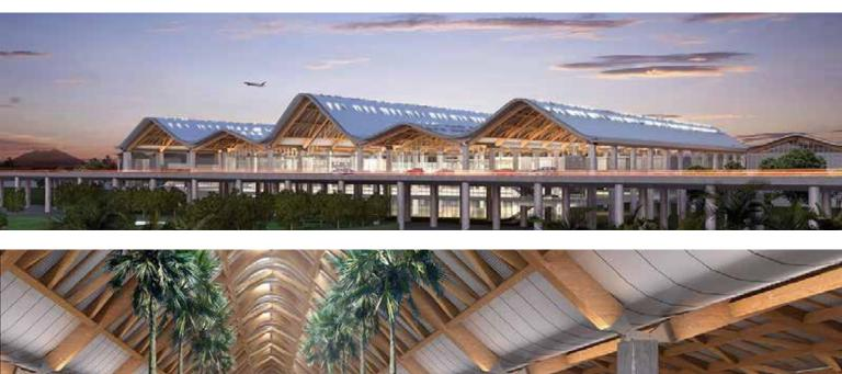
he updated the use of bamboo in modern furniture). But instead of traditional bamboo, the Clark airport project will use glue-laminated (timber) structure—glulam, or structural engineered wood.
