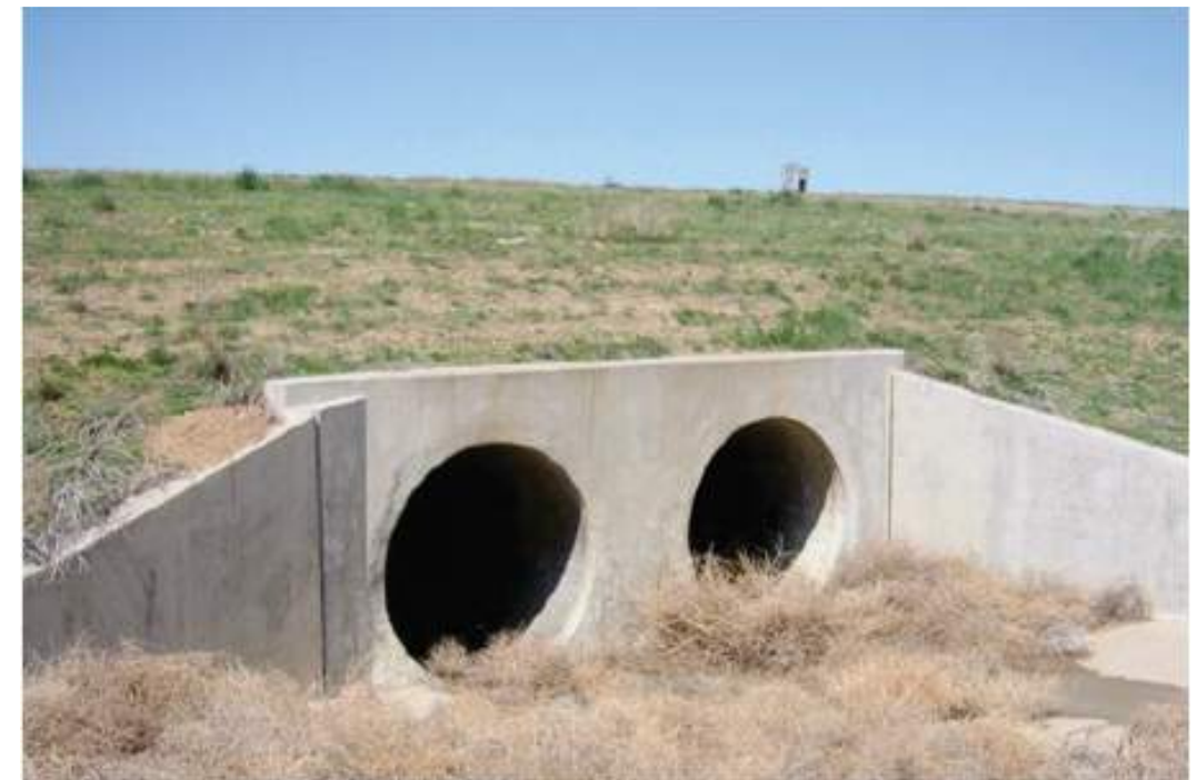
Figure 9.2 Typical Outfall. End of Culvert barrel flush with the headwall
